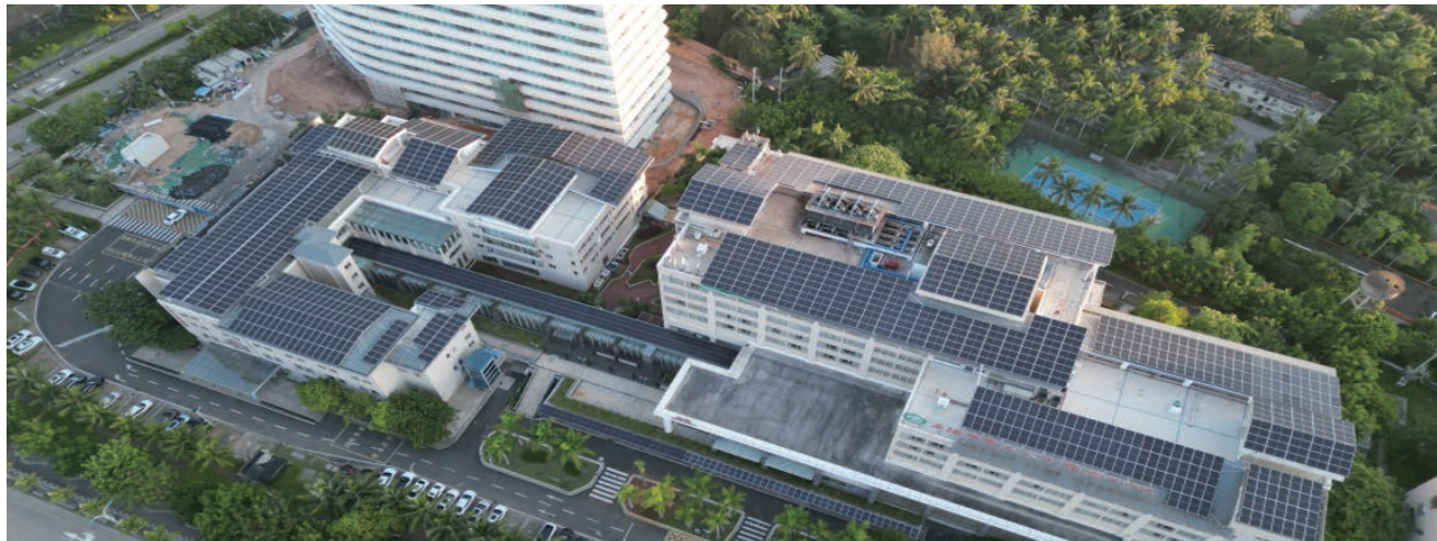
Hainan, China Completed: 2023
